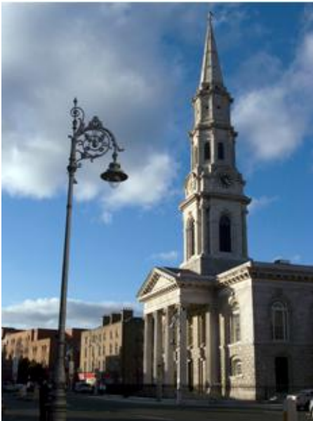
View of Saint George's Church on Hardwicke Place
